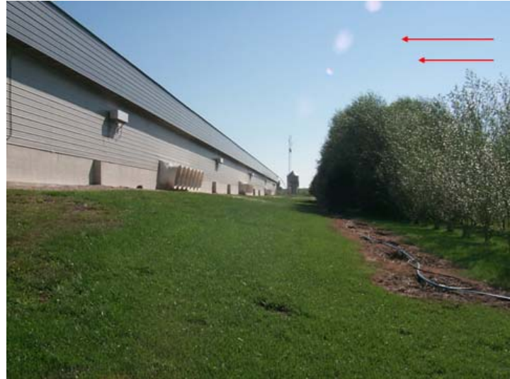
Figure 6. Space between south building and windbreak. Note the 10 m EC tower near the center of the image and the multiple banks of fans.
