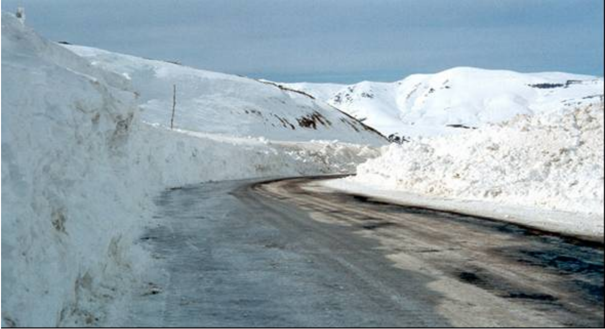
Figure 1.2: A Road with Significant and Recurrent Drifting
