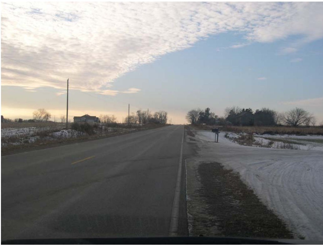
Figure 3.5. Fourth test location, about 2.0 miles west of Highway 1
