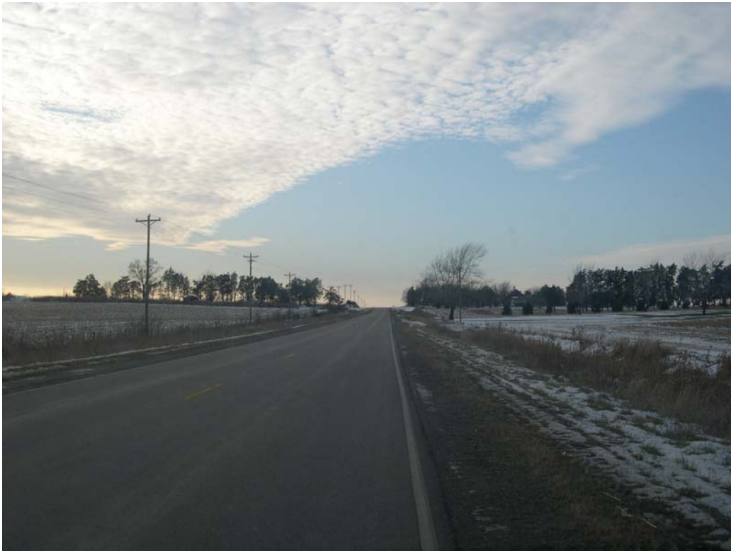
Figure 3.3. Second test location, about 1.0 mile west of Highway 1
